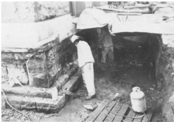
The work sequence for installation of the side beams is shown step-by-step. Here the workman is knocking out pieces of sandstone foundation that have been cut to a 4" depth by the saw.
