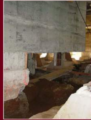
Sequenced Structural Support and Excavation of SW Stair Tower
