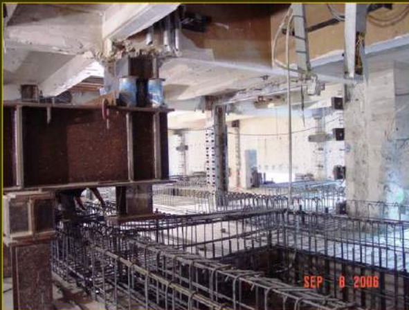
Base Isolators now in Place under Main Dome. Installation of Wood Forms and Rebar for New Concrete Basement Floor
