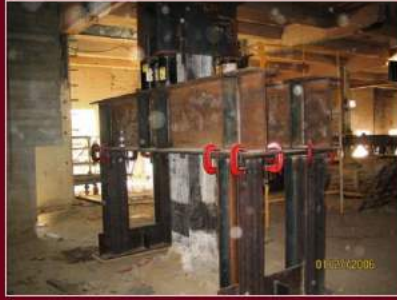
Steel Base Plates Welded to Dome Columns in Preparation for Installation of Seismic Sliders
