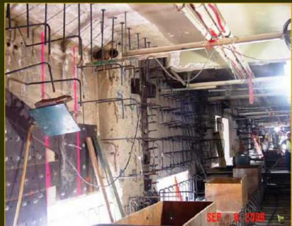
Installation of Reinforcing Steel for Shear Wall at Main Dome Area
