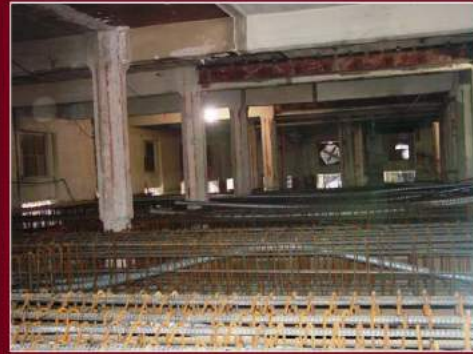
Sequenced Structural Support and Excavation of SW Stair Tower
