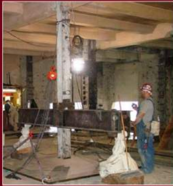
Steel Base Plates Welded to Dome Columns in Preparation for Installation of Seismic Sliders
